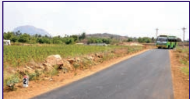
Road Connecting Kidaiyur to Mettur under SCPAR Scheme, Salem District
