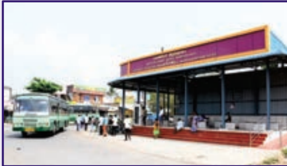
Bus Shelter under MLACDS, at Pudumallavadi Panchayat, Tiruvannamalai District
