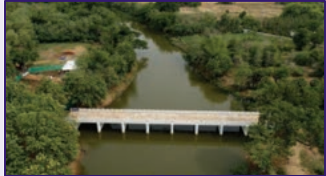
Bridge connecting Sembiyavarambal - Krishnapuram link road under NABARD - RIDF, Thanjavur District
