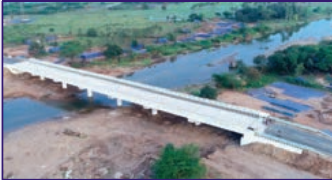
Bridge connecting Kalpoondi to Ladapadi Village under NABARD - RIDF, Tiruvannamalai District
