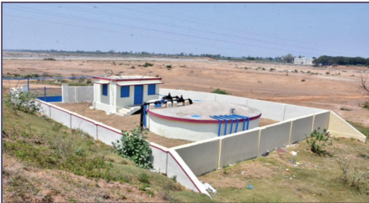
Combined Water Supply Scheme for 9 Panchayats in Panruti and Annagramam Unions of Cuddalore Districts at the cost of Rs.9.21 crore implemented from DMFT Fund
