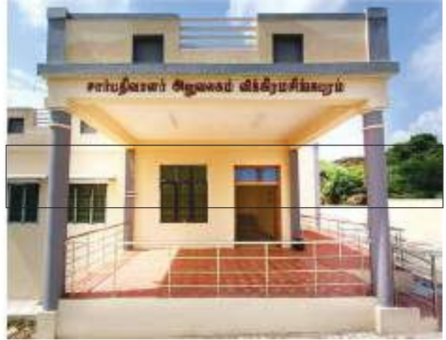
New Sub Registrar Office Building at Vikiramasingsapuram in Tirunelveli Zone.
