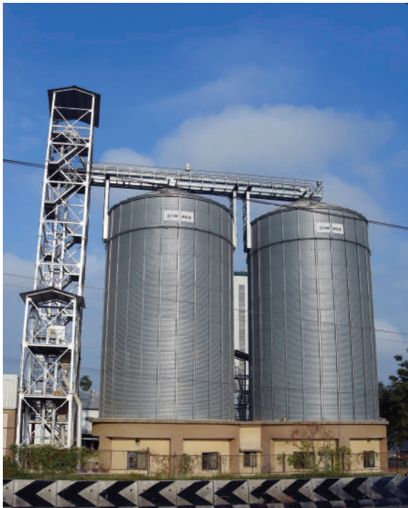
Cattle feed plant with a capacity of 300 MTPD at Erode
