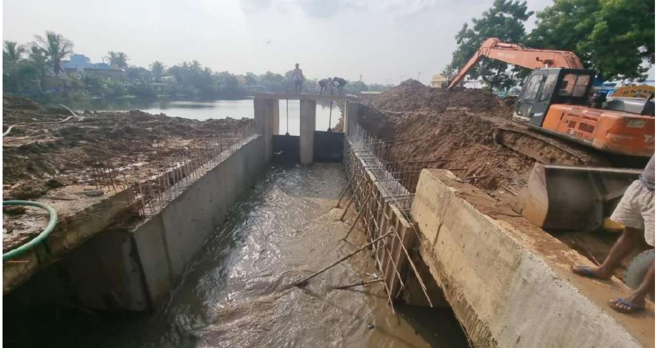
Chennai District- Restoration of bank and deepening of existing tank bed and improvements to its surplus course of Kolathur Tank - Estimate Amount Rs. 7.30 crore - State Fund
