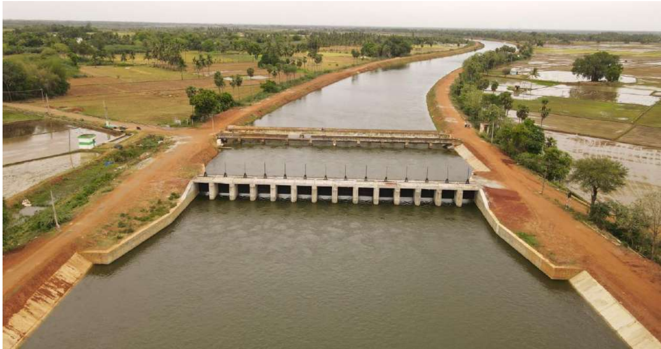
Thanjavur District- Extension, Renovation and Modernisation -Grand Anicut Canal System – New regulator Kuruvadipatti village (Package No -2) – (Estimate Amount Rs.192 crore)- State Fund
