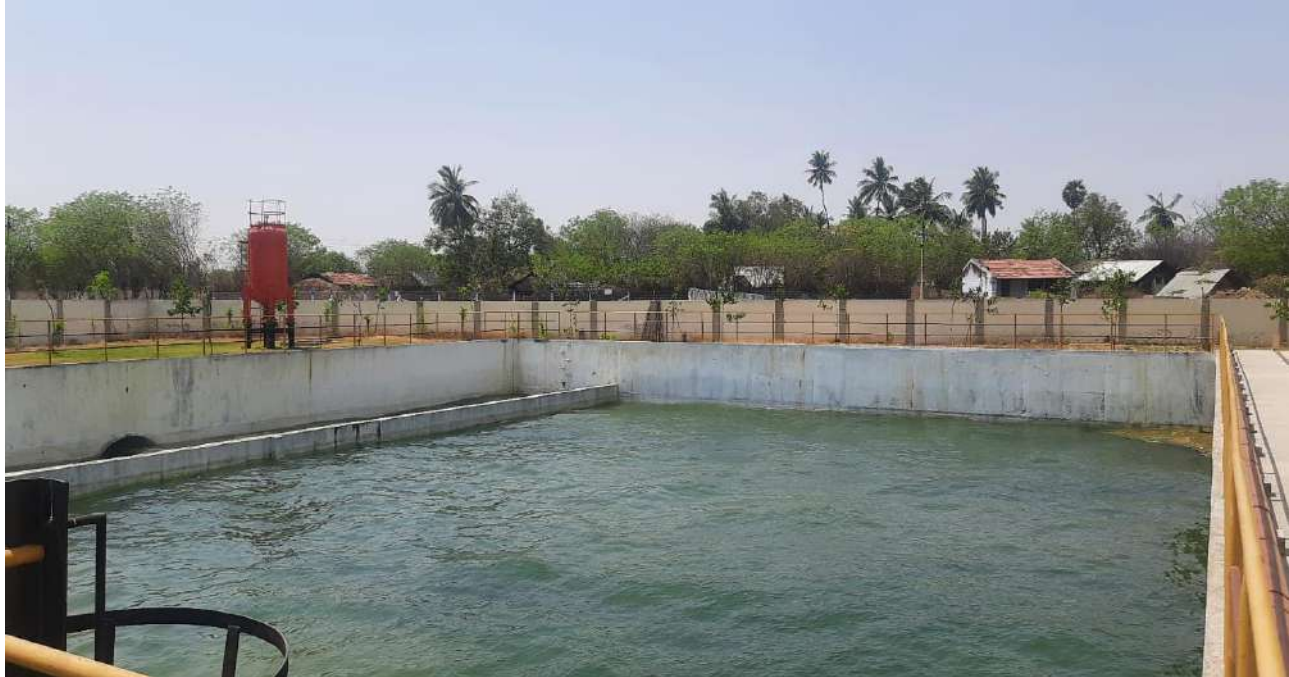
Athikadavu Avinashi Pumping Scheme – Test run from Pumping Station II, NallagoundenPalayam to Pumping Station III, Tiruvachi – Date 26.02.2023
