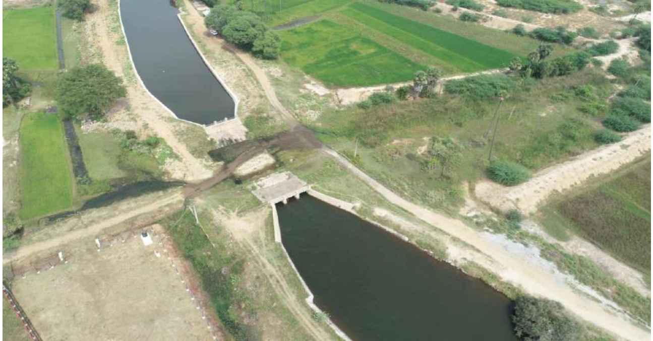
Erode, Tiruppur and Karur District- Extension, Renovation and Modernisation - Protection wall at Mile 64/2 in LBP Main canal (Package No -4) – (Estimate Amount Rs.189.55 crore) - NIDA
