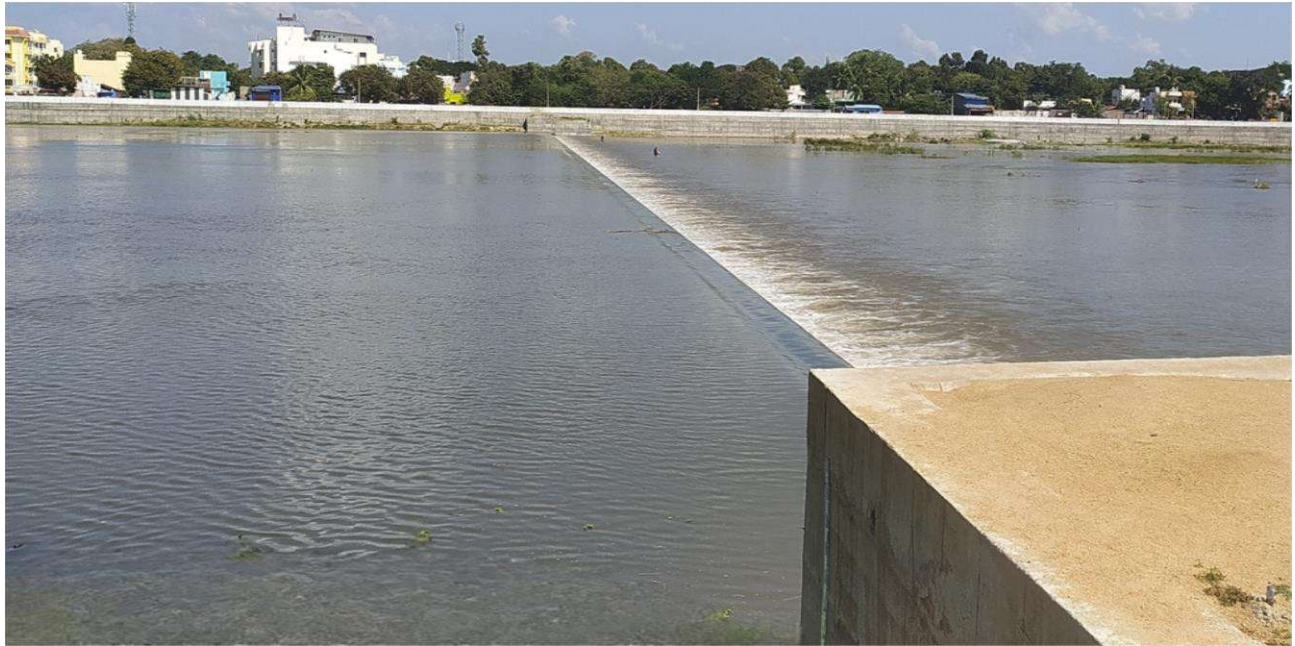
Madurai District - Check Dam and Recharge shaft across the Vaigai River near Aarapalayam Estimate Rs.11.98 Crore – NABARD Fund
