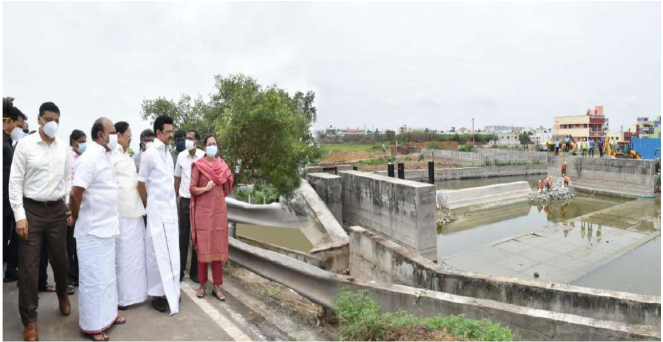
Kancheepuram District- Hon'ble Chief Minsiter Visit of the work for Improvements on Porur Tank Surplus Course and Regulator Arrangements
