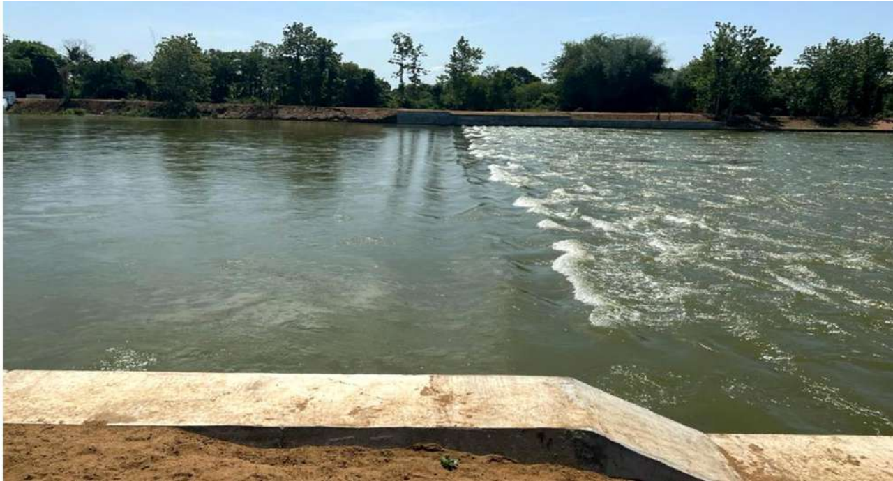
Thanjavur District - Grade wall across Vennar River at LS 85.180 Km in Ivelithottam Village – (Estimate Rs.5.856 crore) - NABARD
