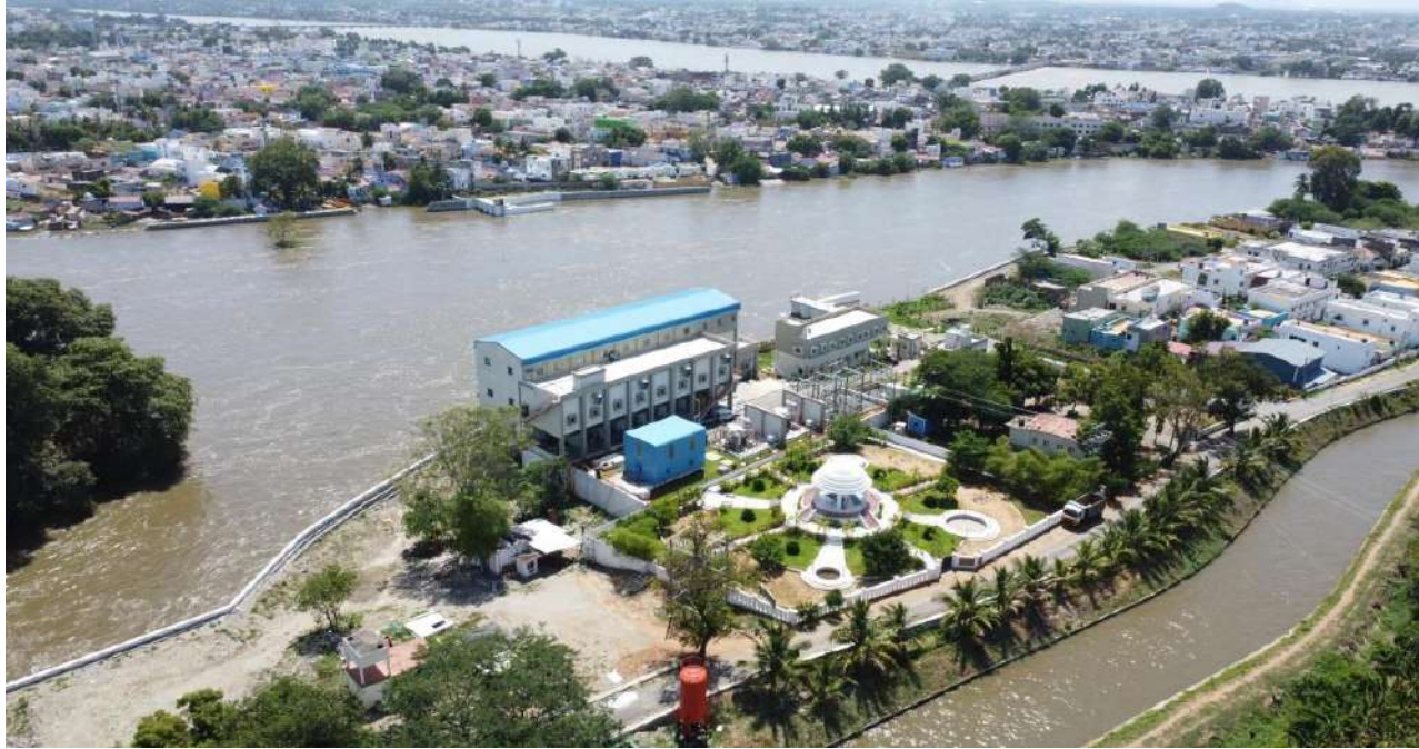
Erode District – Bhavani Taluk, Athikadavu Avinashi Pumping Scheme Pumping Station I at Bhavani– Estimate Amount Rs.1756.88 Crore – State Fund.
