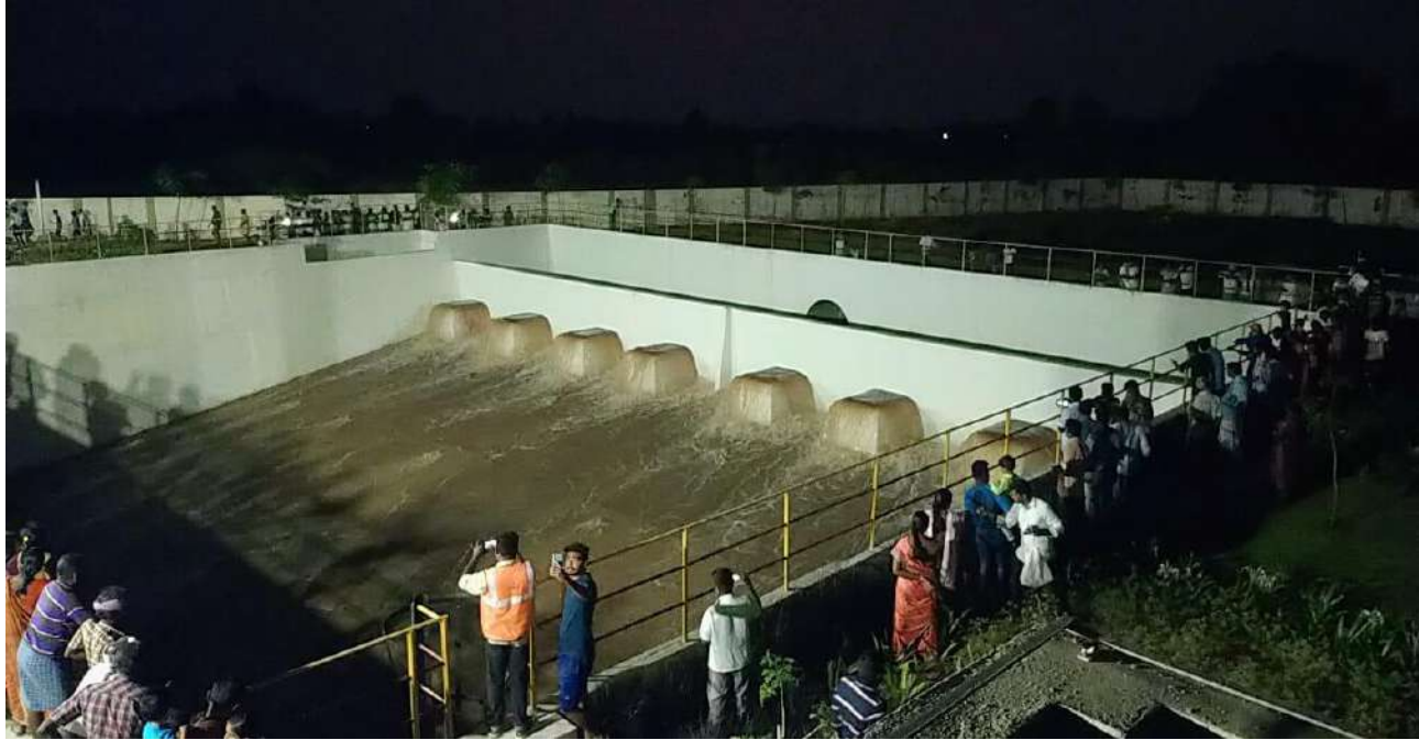
Athikadavu Avinashi Pumping Scheme – Test run from Pumping Station III, Tiruvachi to Pumping Station IV, Polanaickenpalayam– Date 04.03.2023
