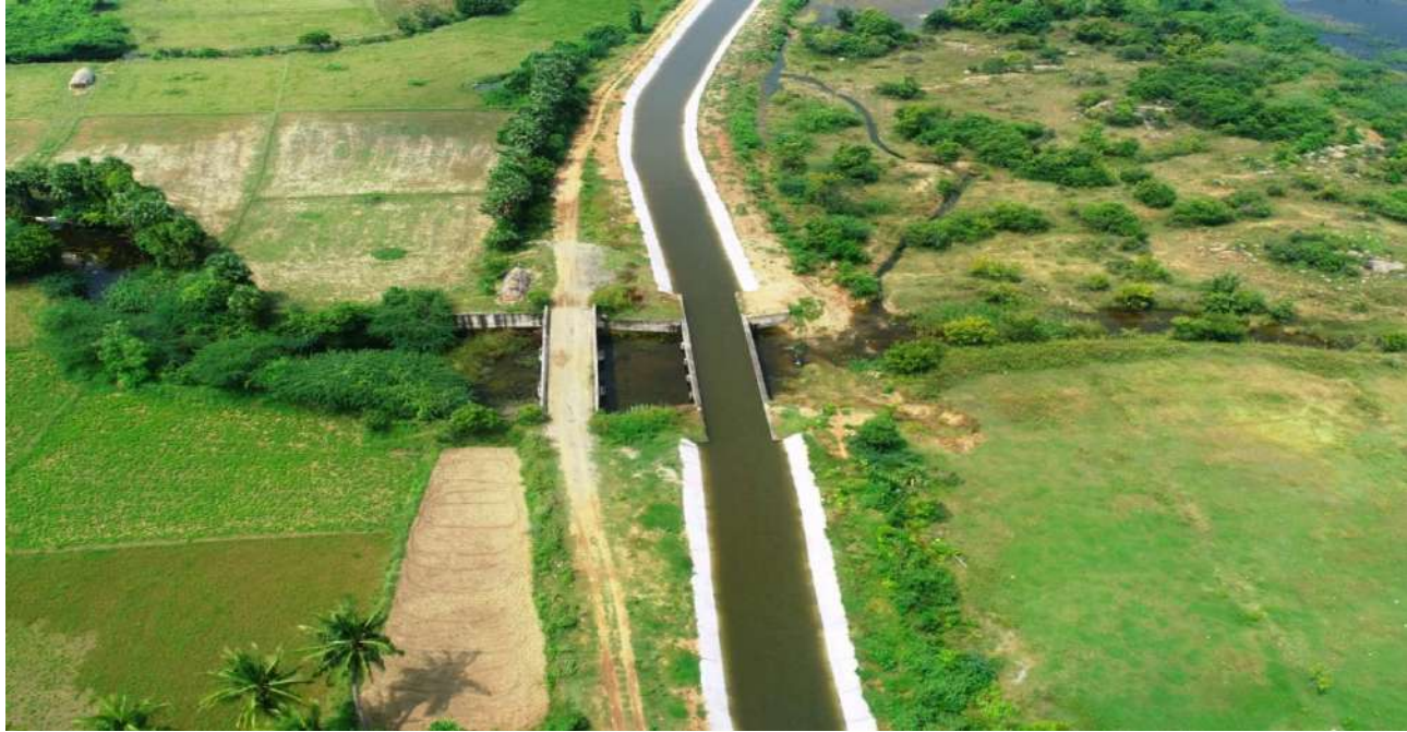
Thiruvannamalai District - Rehabilitation and Improvements to the Nandhan Channel form L.S. 0 Km to 12.40 Km in Thiruvannamalai and Kilpennathur Taluk - Estimate Amount Rs. 7.26 crore – NABARD Fund
