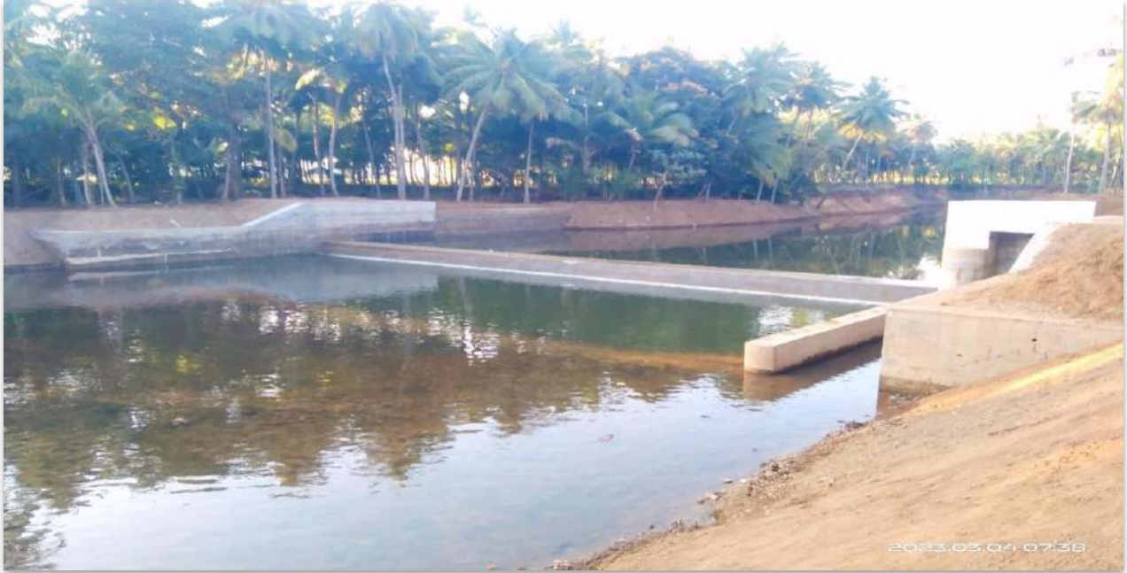
Theni District - Check dam across Manjalar River near Genguvarpatti village Estimate Rs.2.36 crore - State Fund
