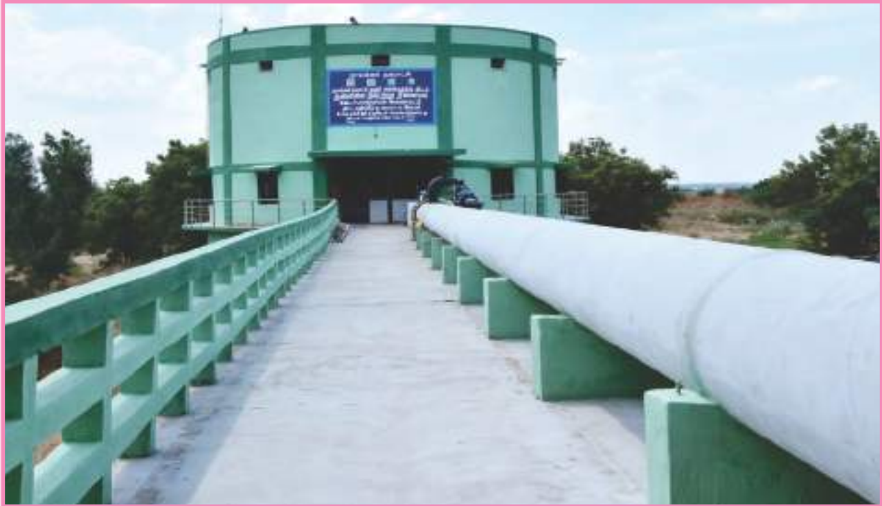
Head works at Jaderpalayam, Water supply improvement scheme to Namakkal municipality in Namakkal district
