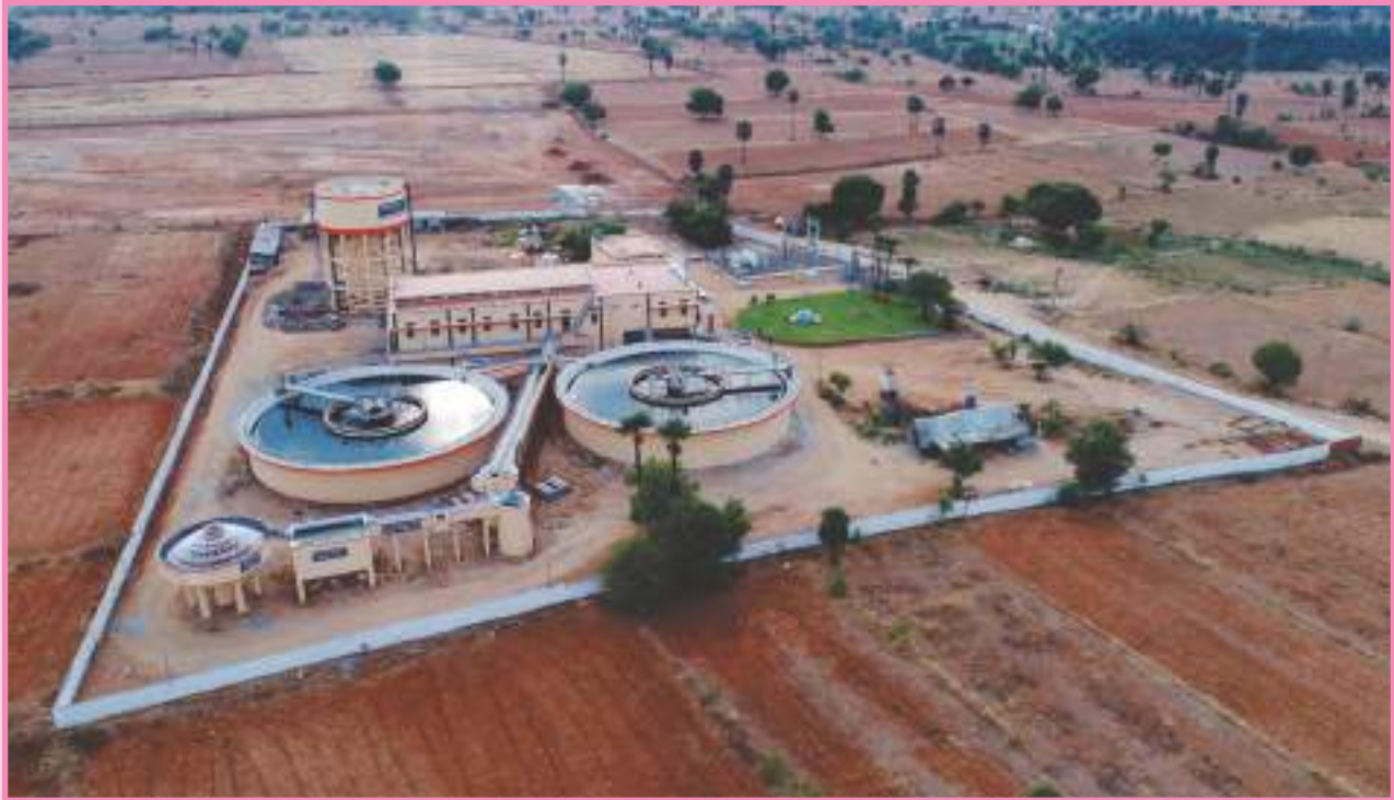
17.23 MLD capacity water treatment plant, constructed under CWSS to Perundurai and 7 other town panchayats including 547 rural habitations in Erode and Tiruppur districts.
