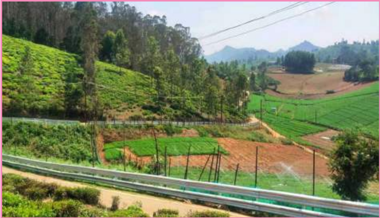
Provision of crash barrier along the road from Muttinadu to Kolanimattam in Adigaratty town panchayat (The Nilgiris district), Scheme : Kalaingar Nagarapura Mempattu Thittam; Project cost : Rs. 45.20 lakh
