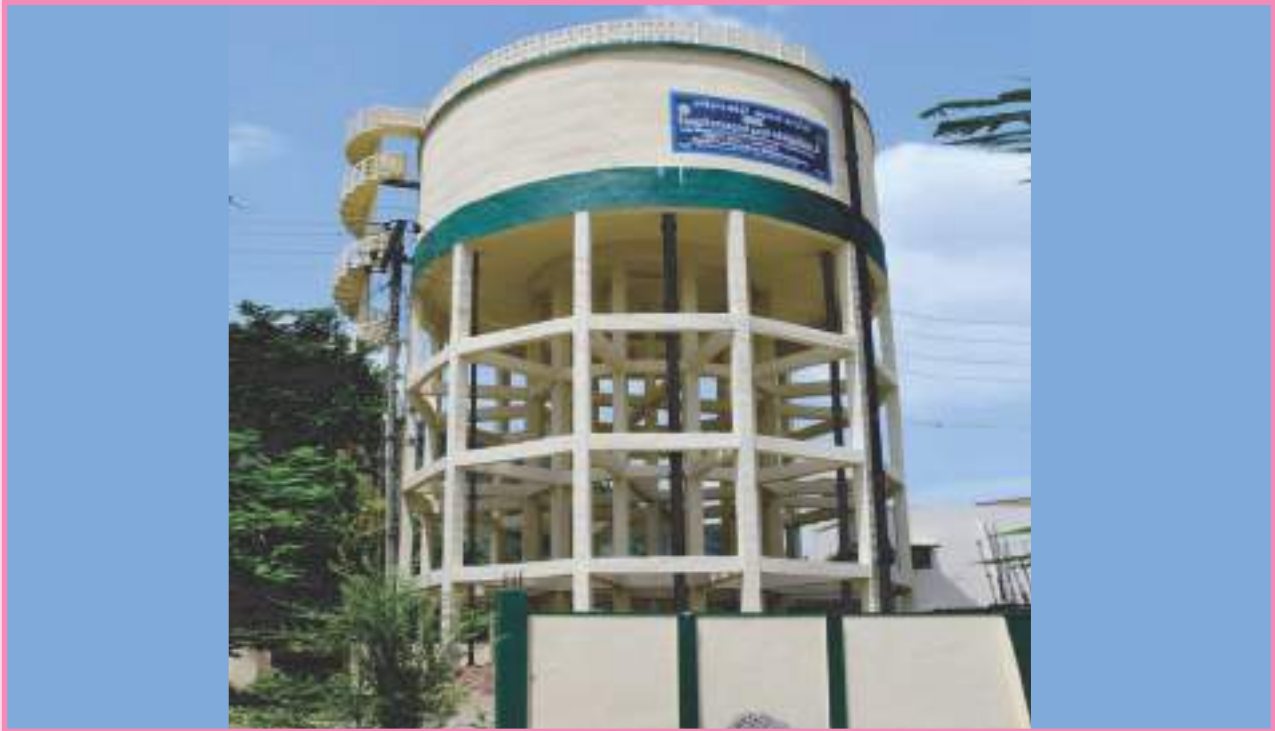
10 lakh litre capacity overhead tank constructed under water supply improvement scheme to Vellore corporation
