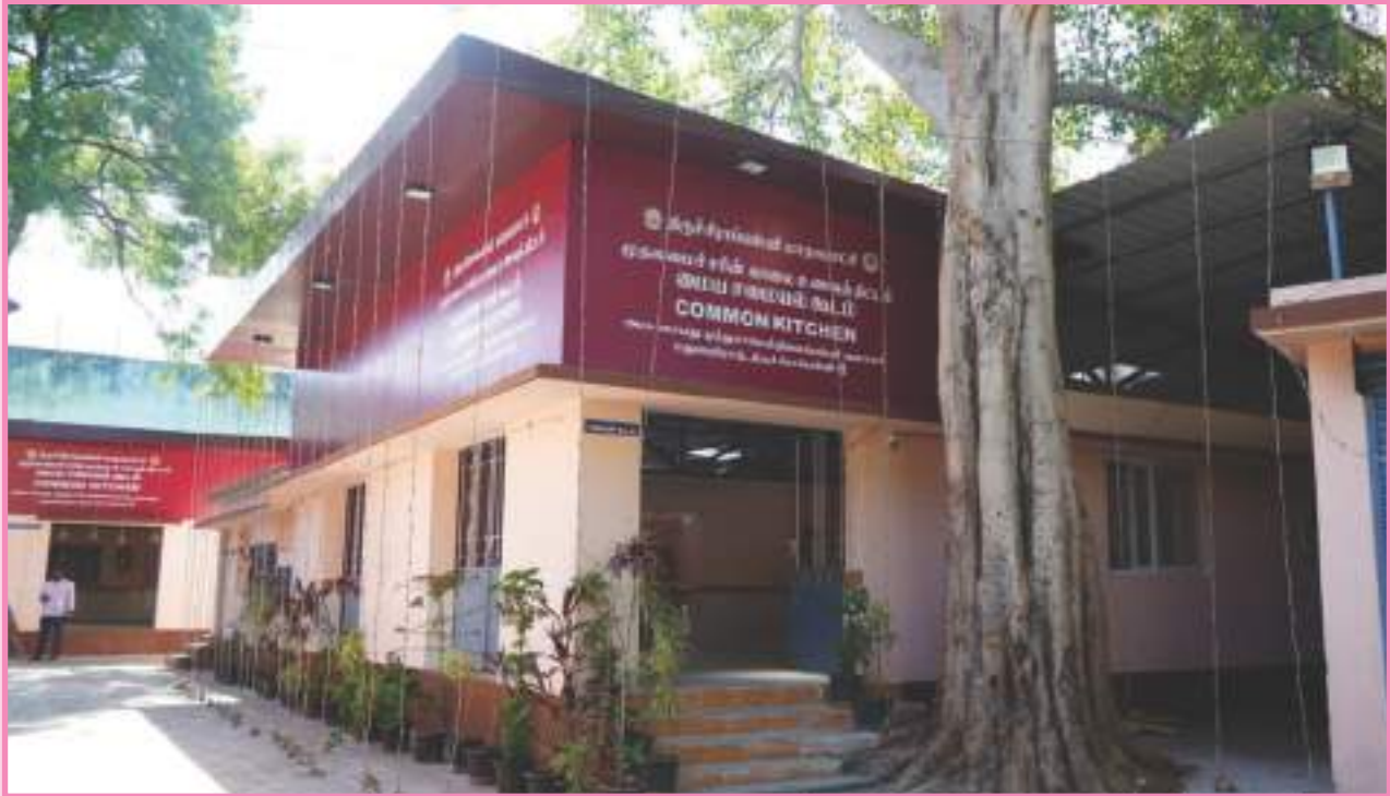
Construction of common kitchen in Tiruchirappalli corporation, Scheme : Chief Minister's Breakfast Scheme; Project cost : Rs. 1.29 crore
