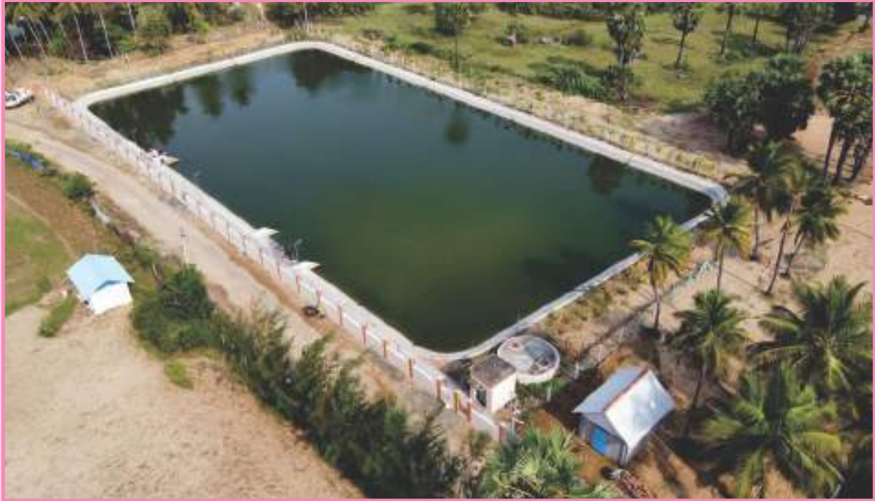
Rejuvenation of Vanadurgai Amman Kulam in Vedaranyam municipality (Nagapattinam district), Scheme : Kalaignar Nagarapura Mempattu Thittam; Project cost : Rs. 57.80 lakh
