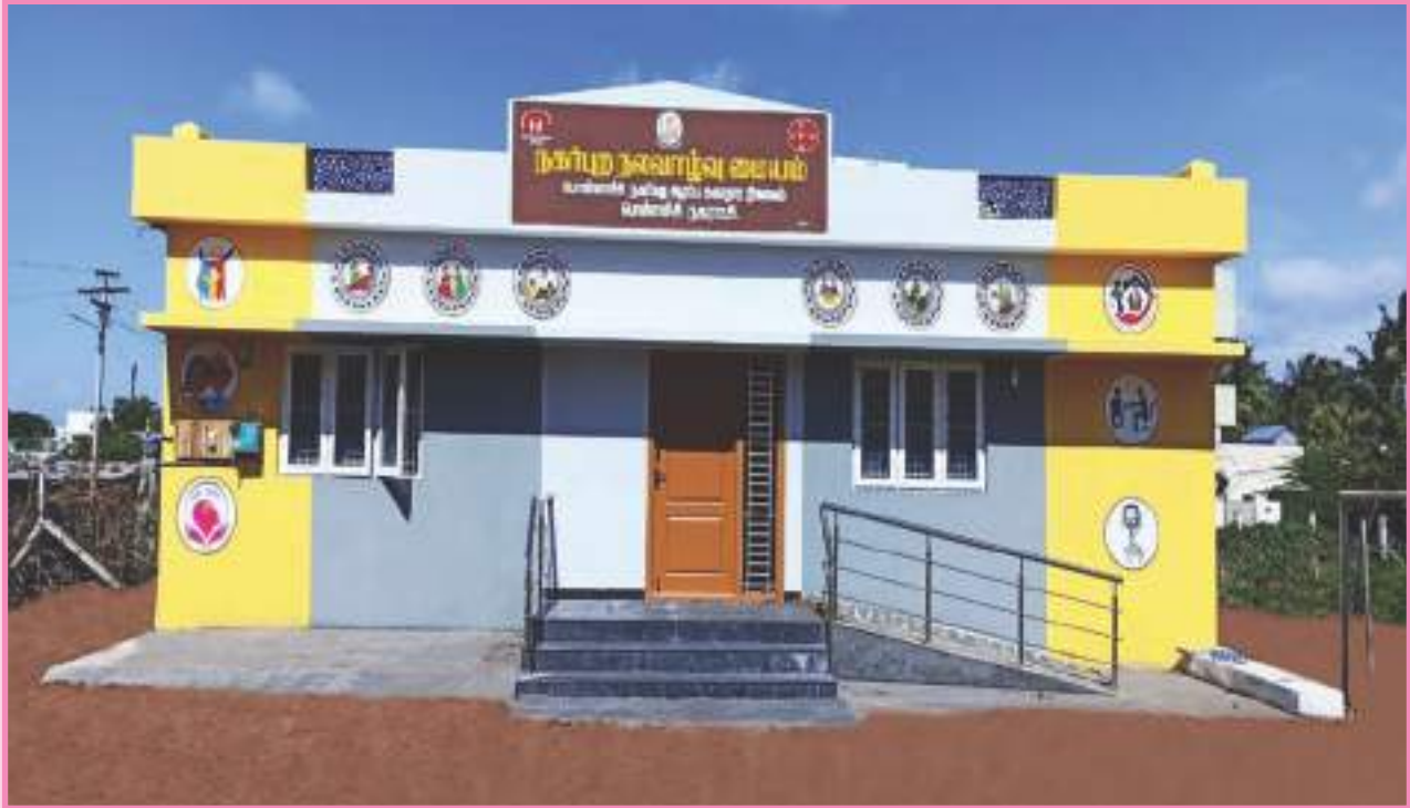
Construction of urban health & wellness centre in Pollachi municipality, Scheme : 15th Finance Commission Grant; Project cost : Rs. 25.00 lakh
