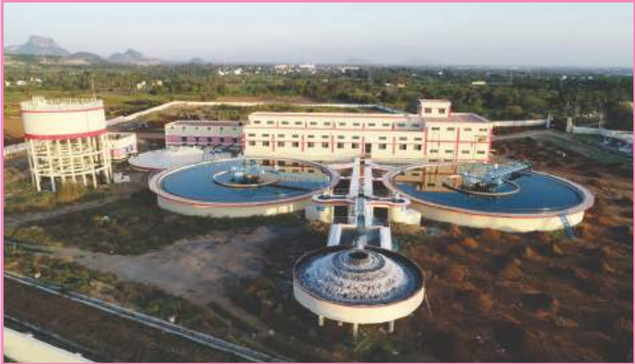
25.51 MLD capacity water treatment plant, constructed under CWSS to Sankari, Alampalayam and Padaveedu town panchayats and 669 rural habitations in Pallipalayam and Tiruchengode unions in Namakkal and Salem districts
