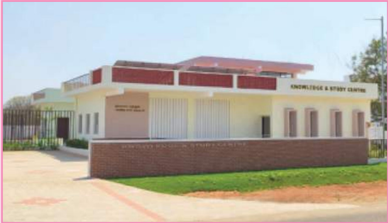
Construction of library cum knowledge centre building in Namakkal municipality, Scheme : Kalaignar Nagarpura Mempattu Thittam; Project cost : Rs. 2.00 crore
