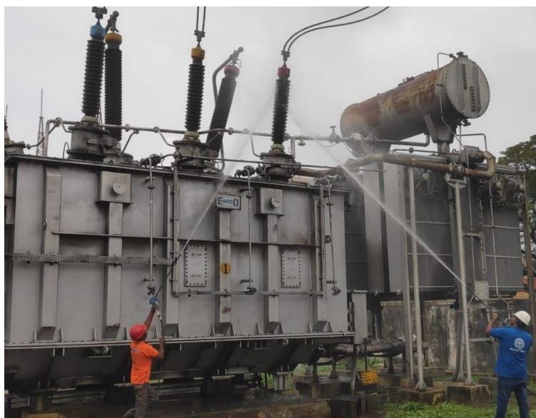
Hotline water washing at 230 kV Kilpauk SS
