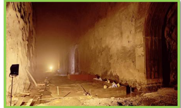
Transformer Cavern – Mud Mat laying work in progress
