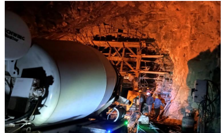
TRT – Tail Race Tunnel Overt lining work in progress
