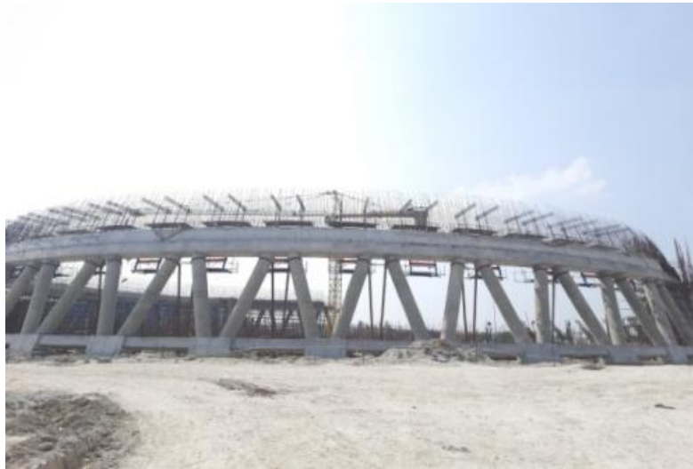
Natural Draught Cooling Tower -01 CONSTRUCTION
