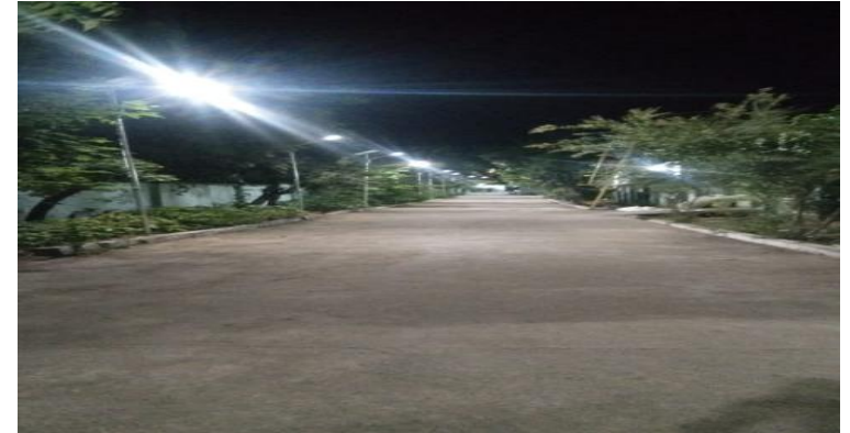
Solar Powered Street Lights, TAMPCOL, Chennai
