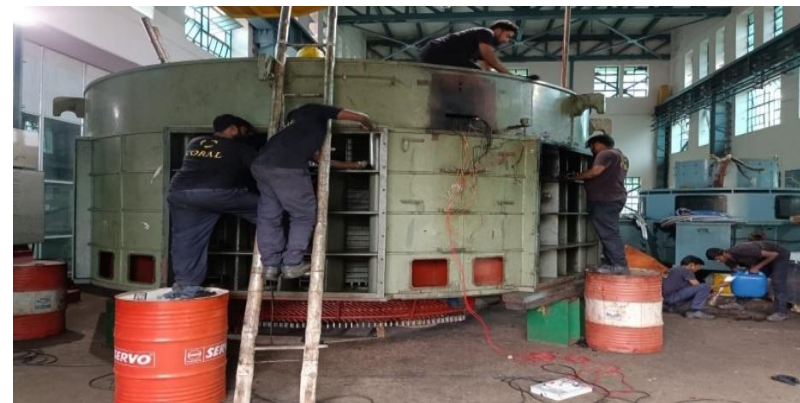
Stator coils rectification work at Kodayar PH-II
