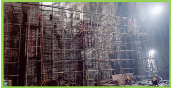
Service Bay – Column Concreting work completed upto Elevation 1939.20–12Nos
