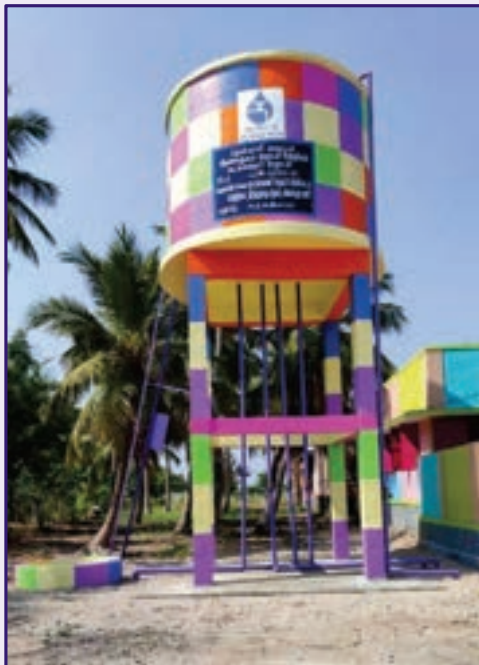
OHT at Kadanganeri Panchayat, Tenkasi District
