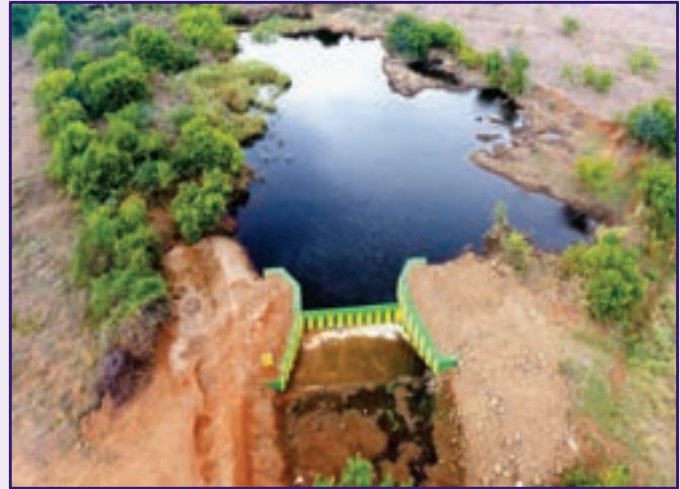
Cement Concrete Check Dam at Thalavaipattinam Panchayat, Tiruppur District
