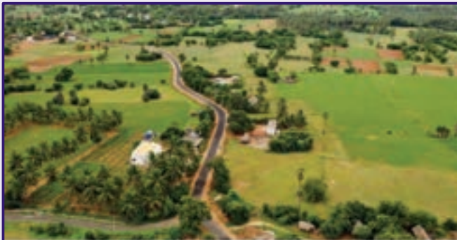
Road Connecting Chittampalayam road to Thudupathi under PMGSY Scheme, Erode District
