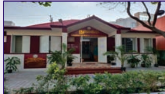
Renovated AGAMT Library, at Mannivakkam Panchayat, Chengalpattu District
