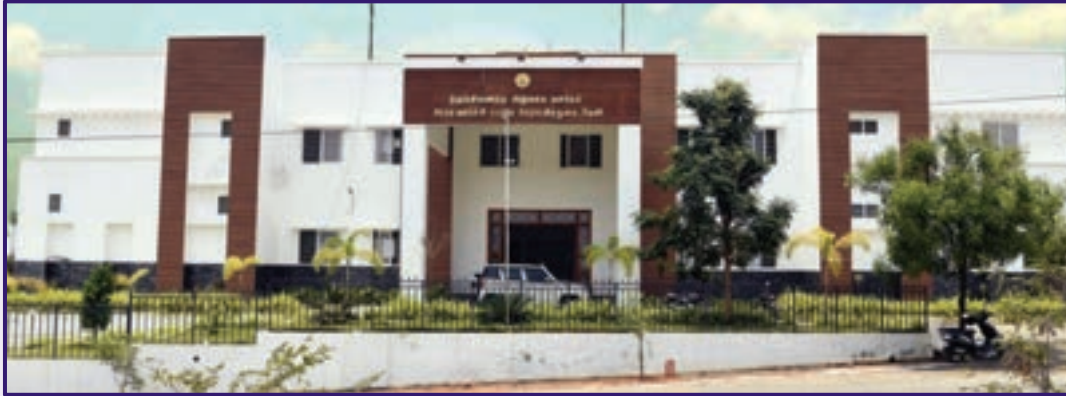
Integrated Office Complex for Rural Development and Panchayat Raj under Scheme Component of Pooled Assigned Revenue Scheme, Theni District
