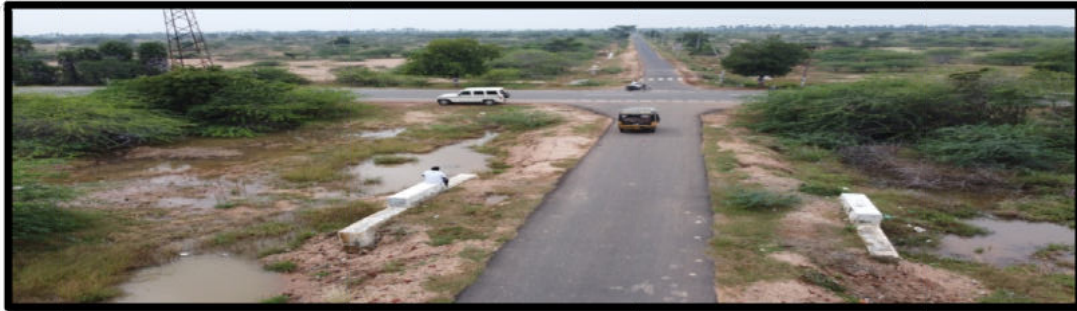
Before Road Safety Work
