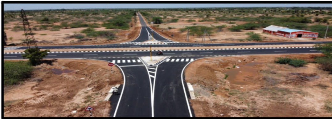
After Road Safety Work
