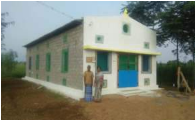
Silkworm Rearing Shed Constructed under MGNREGS
