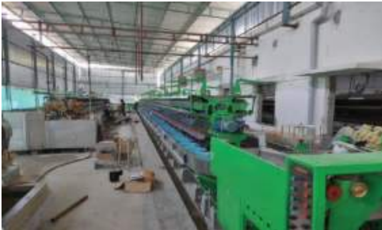
Automatic Dupion Silk Reeling Machine Unit, Udumalpet
