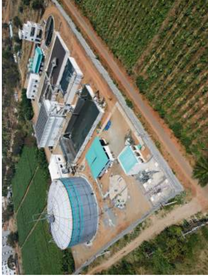
Aerial view of Sewage Treatment Plant at an Educational Institution in Erode
