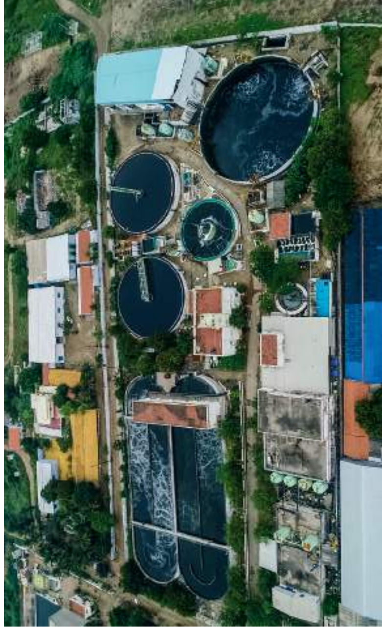
Aerial view of textile CETP at Tiruppur
