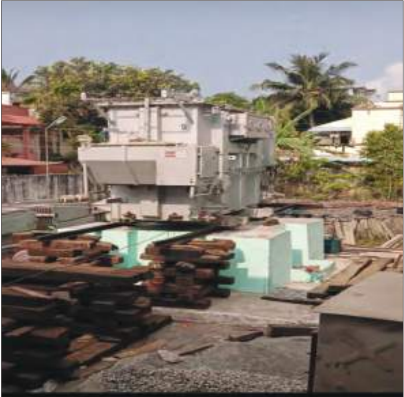
Periyar Nagar 33/11kV SS-, Perambur Plinth Heightening
