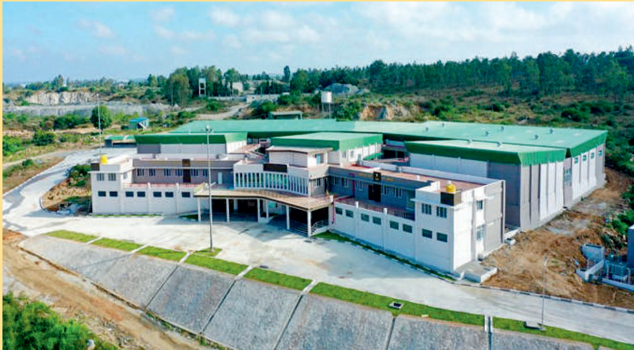
Construction of International Flower Auction Centre in Hosur with facilities to store 2.50 Lakh flower stems at refrigerated warehouse, Auction Centre, Grading Centre, Traders Centre, Cold Storage Unit of 2,000 tonnes capacity, Conference Hall and 16 Retail Outlets.
