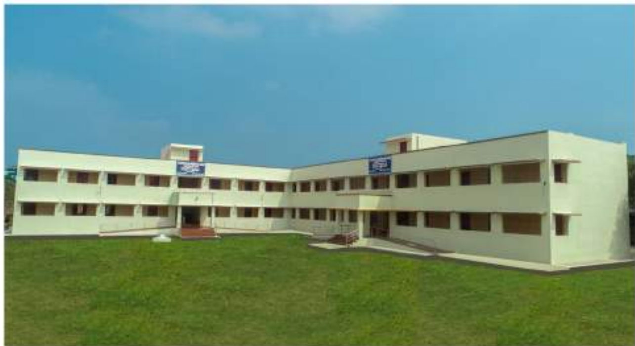
The newly constructed Higher Secondary School at Kilambakkam in Chengalpet District, (Estimate Amount: Rs. 279.90 Lakh).
