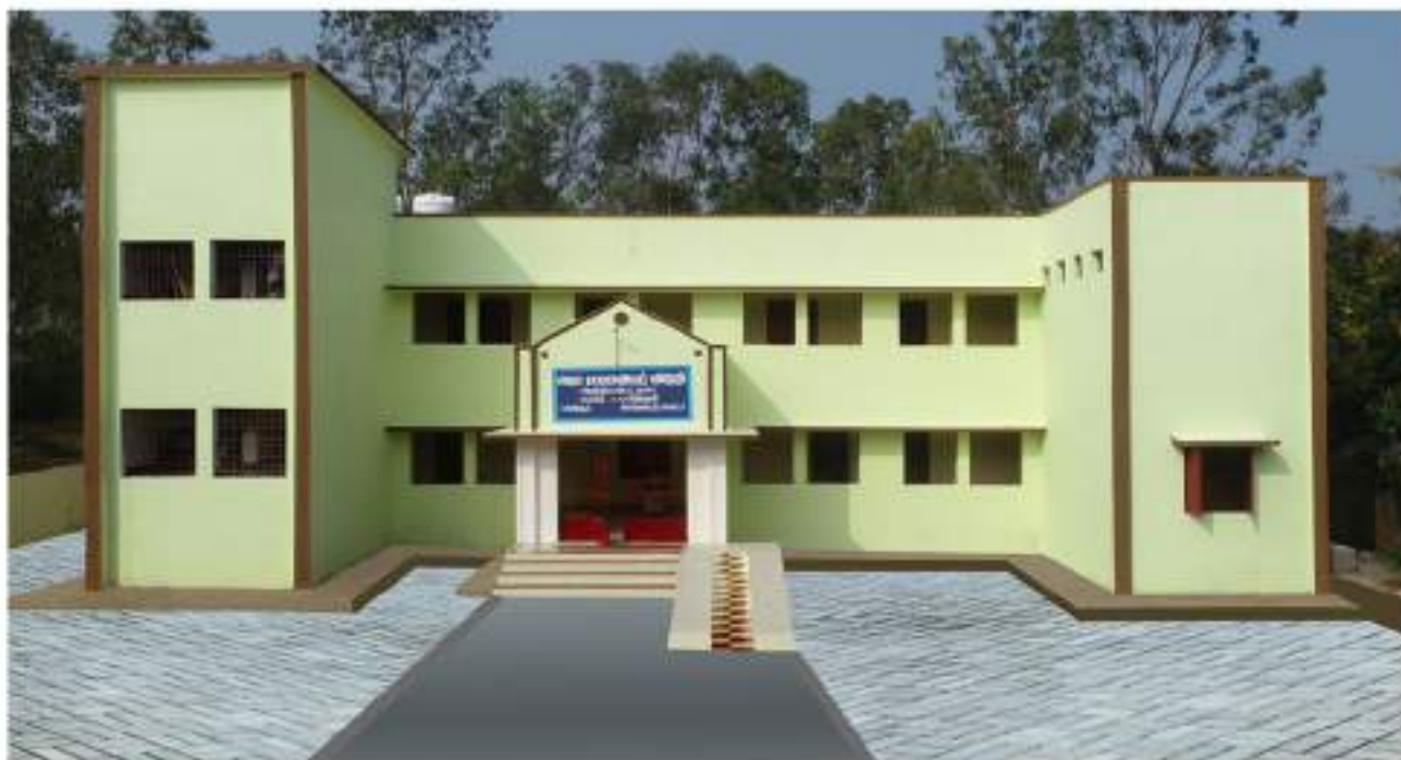
The newly constructed Adidravidar Welfare School Girls Hostel Building at Pounjur in Chengalpeta District (Estimate Amount: Rs. 111.03 Lakh).
