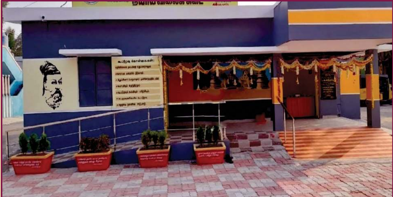
New building of Ganesanagar Fair Price Shop run by Kanchipuram District Consumer Cooperative Wholesale Store in Kanchipuram District.
