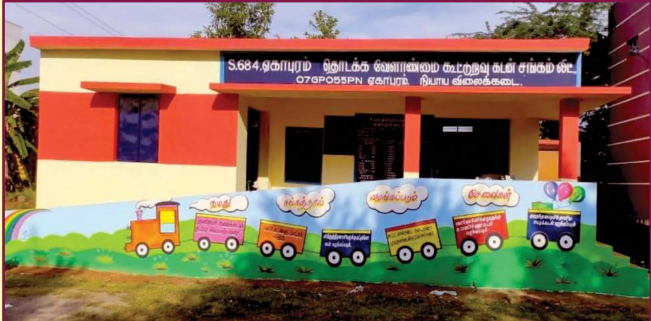
New look of Fair Price Shop of Salem District Ekapuram Primary Agriculture Co-operative Credit Society under Fair Price Shops Facelifting Programme.
