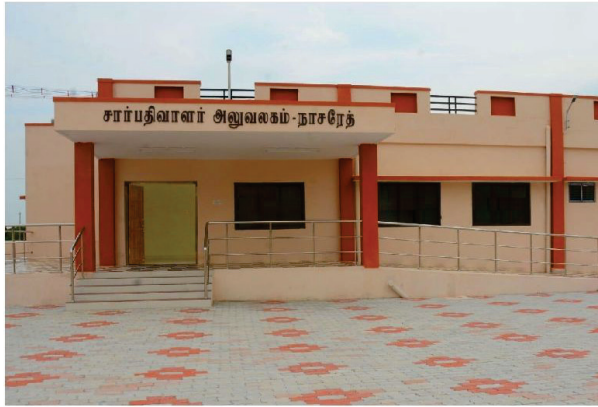
New Sub Registrar Office Building at Nazareth, Tirunelveli Zone.
